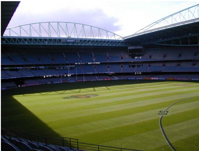
Figure 2 Colonial Stadium with its retractable roof open. Each level sits above the previous one providing a compact stadium with proximal views for all patrons.
