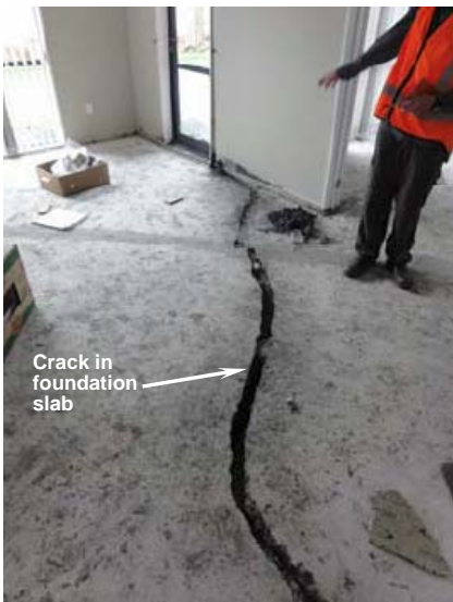
(c) Cracked foundation slab due to lateral spreading
