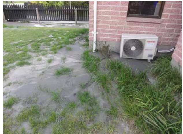
(a) Sand ejecta at the perimeter of house foundations
