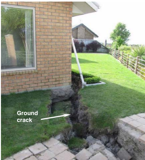
(b) Lateral spreading cracks in foundation soils
