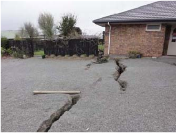
(a) Lateral spreading crack running through residential house
