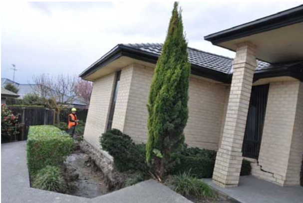
(b) Excessive tilt and uplift of foundations due to lateral spreading displacements of about 1.5 m
