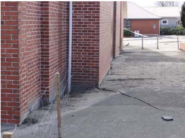
(c) Evidence of liquefaction in foundation soils (view looking north; east side of building)
