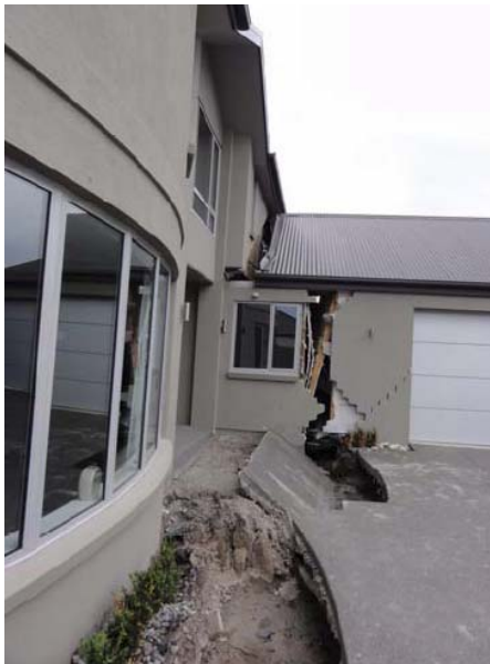
(c) Severe damage to residential house due to lateral spreading displacements of about 1.5 m
