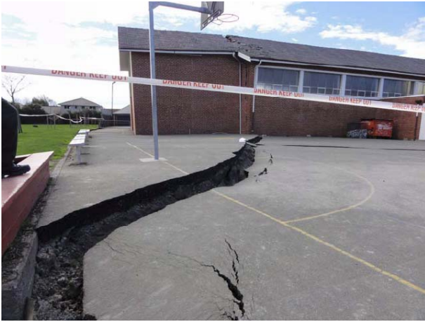
(a) 50-90 cm wide ground crack with a vertical offset of 33 cm at its maximum (view looking north)
