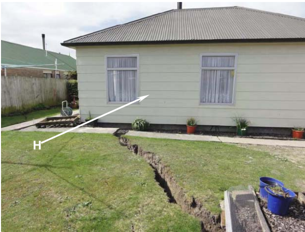
(b) Lateral spreading crack running through residential house
