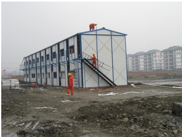
Figure 5: Double storey prefabricated units
