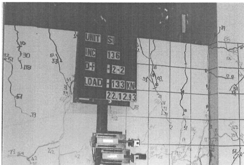
Fig. 5.1b Cracking in the Splice Region at \mu = -2/2 .
