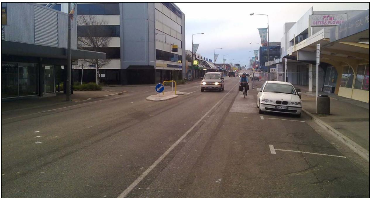
**Figure 2: Mid-Block Cycle Lanes next to kerbside (left) and parking (right)**
