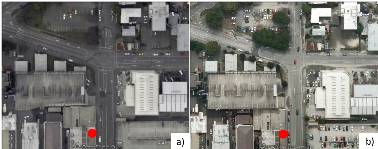
Figure 6. CHHC liquefaction surface manifestation a) Darfield earthquake; b) Christchurch earthquake
