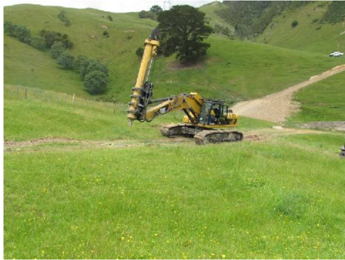
Figure 3: A track mounted drilling rig climbs a temporary access track
