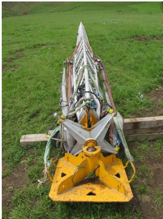
Figure 6: The gin pole used by a UK subcontractor to erect tower 157
