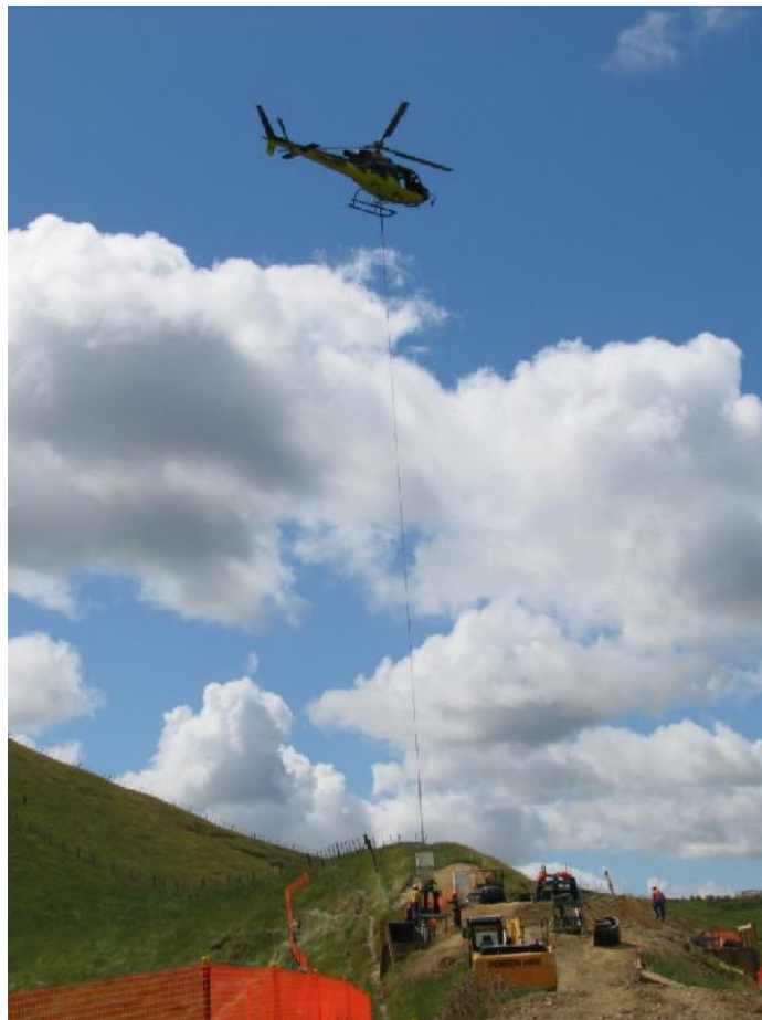
Figure 4: A bucket of concrete is delivered to site for foundation works
