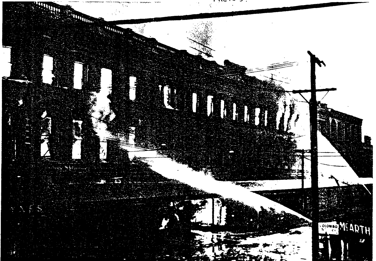
The Cashel Street frontage, with water flooding the street as hoses are played on the windows from which many people trapped in the blazing building were rescued. The heat was so intense that in parts of the building the Oamaru stone facing turned into lime.
