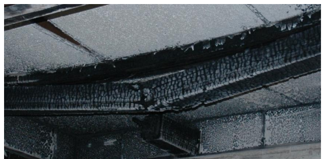
Figure 21: Test 2 beam after the test.
