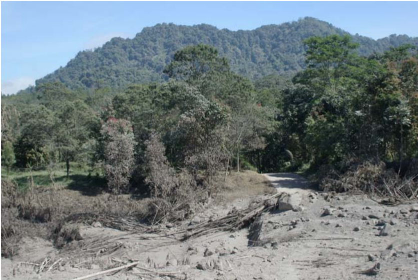
Figure 18 Road close to Kaliadem partially covered by debris from 14 June flows (note sharp boundaries)
