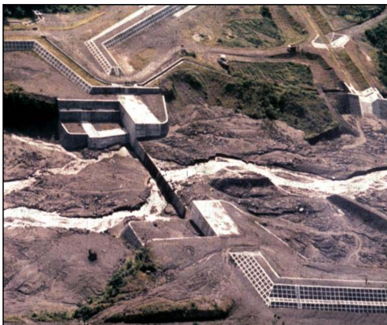
Figure 35 Sabo dam in Indonesia
