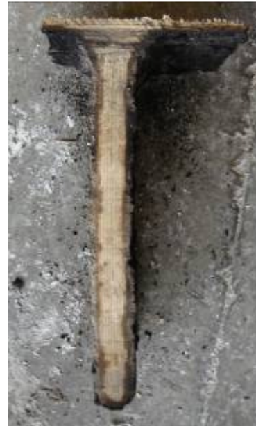
Figure 6: Residual section of the beam floor after 31 minutes fire exposure (7 minutes additional charring)
