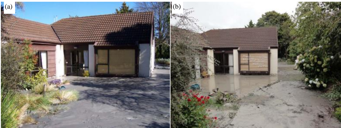
Figure 20: Illustration of a house in Kaiapoi which sustained liquefaction in both the (a) 4 th September 2010 Darfield; and (b) 22 February 2011 Christchurch earthquakes.
