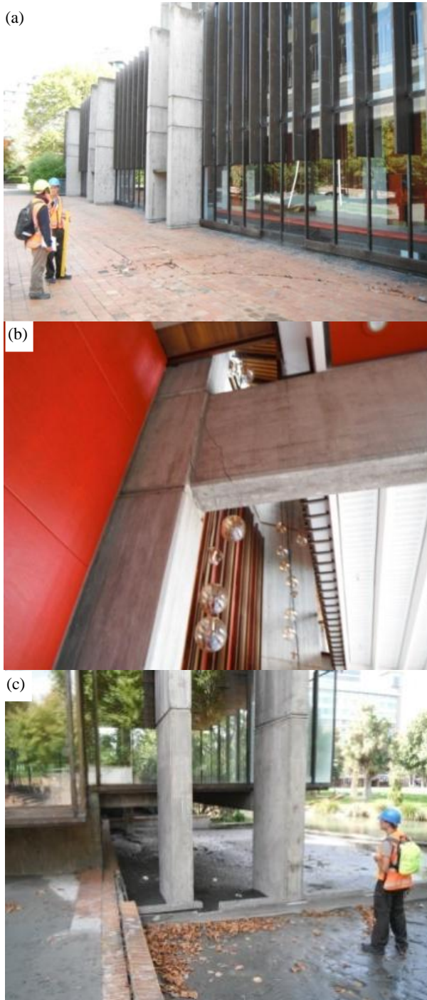
Figure 14: Town Hall auditorium and adjacent dining facility undergoing significant liquefaction-induced differential settlement and lateral movements [7].
