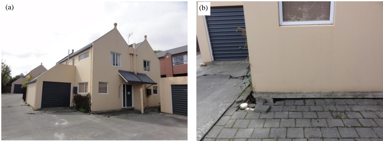
Figure 11: Duplex housing complex: (a) looking north at centre building, and (b) close-up of ground settlement next to centre building [7].
