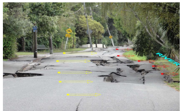
Figure 24: Lateral spreading toward the Avon River.
