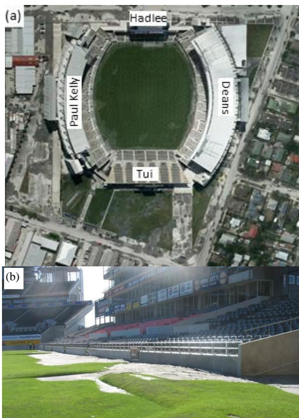
Figure 33: (a) Aerial photo of AMI Stadium indicating liquefaction damage; and (b) Liquefaction damage to the stadium field.
