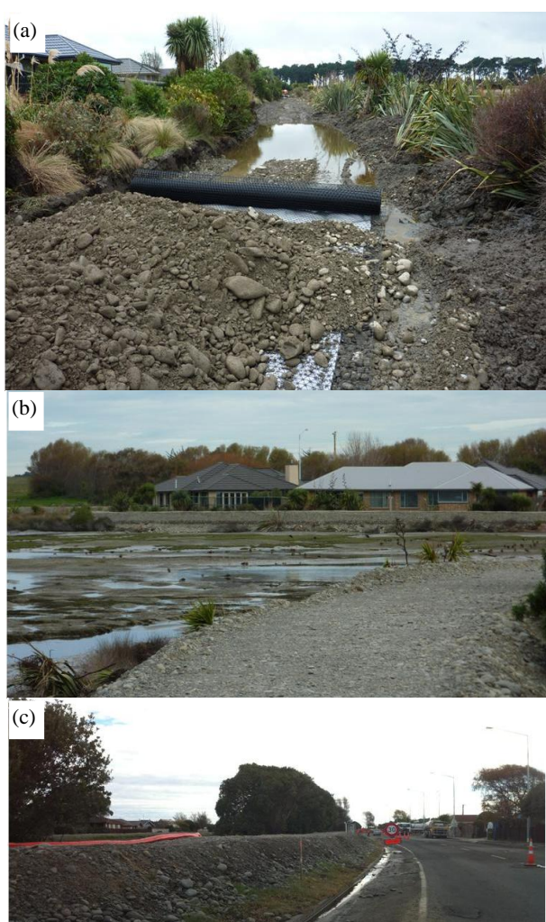
Figure 25: (a) Fill material used for construction and geogrid/liner for temporary stop banks; (b) position of residences below temporary stop banks in Bexley wetland; and (c) stop bank construction along New Brighton Rd.
