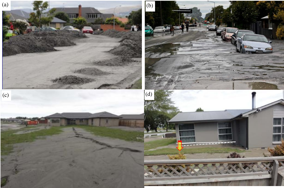
Figure 19: Typical manifestation of liquefaction in residential areas.
