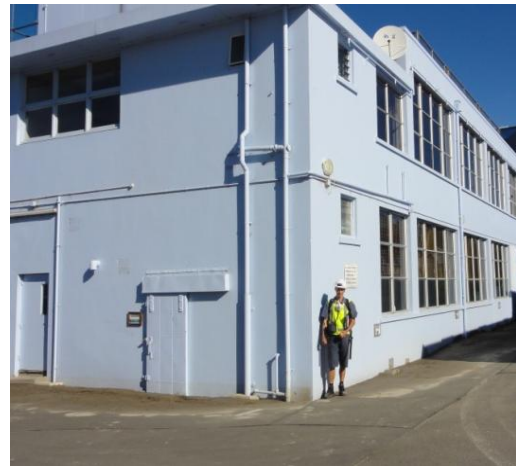
Figure 12: Two-storey building that underwent liquefaction-induced punching movements [7].
