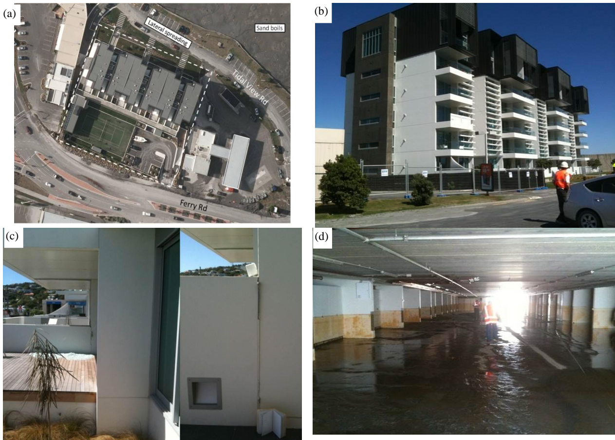
Figure 32: (a) Aerial view of Ferrymead apartment building indicating surrounding ejected material; and (b) south-west looking view of the apartments; (c) separation of walls on the north side of the building, including sloping of the separation walls and shattered glass panels, and compression of caulk at top of expansion joint; and (d) the basement parking garage. Note the high water mark on the walls.
