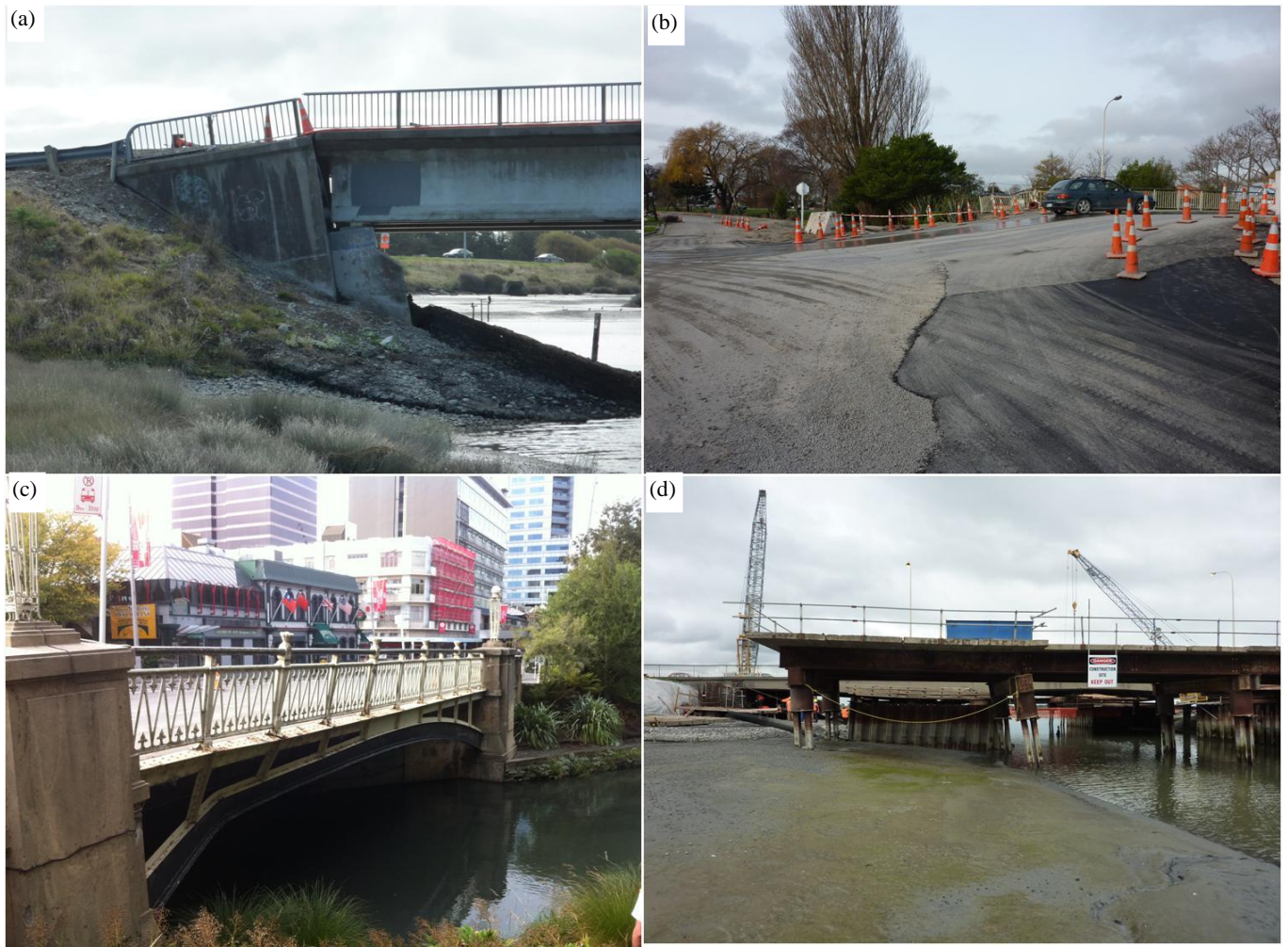
Figure 26: Summary of bridge damage: (a) back-rotation and settlement of the western abutment of South Brighton bridge; (b) settlement of the northern approach of Gayhurst Road bridge following the June 13 2011 earthquake; (c) abutment back-rotation and buckling of the steel arches of Colombo Street bridge; and (d) movement of temporary construction platform for Ferrymead bridge due to lateral spreading.
