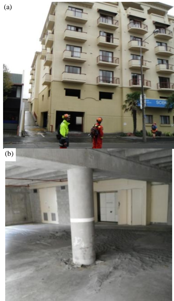
Figure 15: Building in area of significant liquefaction that displays negligible to minor differential settlement or punching settlement [7].
