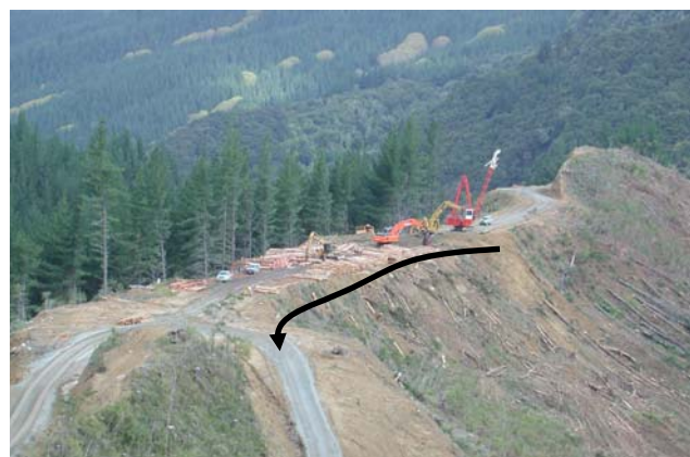
Figure 3: Arrow overlaid on cable landing showing linear flow of production.
