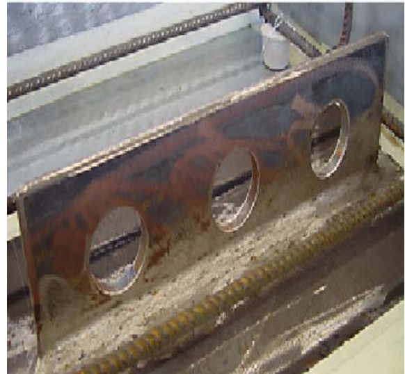
Fig. 2-8. “Perfobond” perforated steel plates (Miotto and Dias, 2008)
