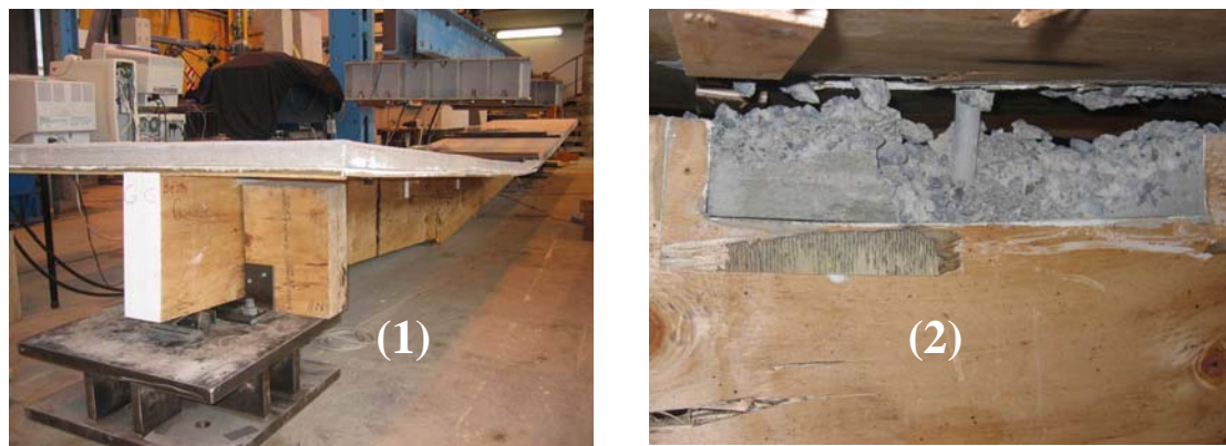
Fig. 5-7. Different types of failure mechanisms detected in the composite beams: (1) fracture in tension of LVL; (2) failure for concrete shear and crushing in 300 mm rectangular notch coach connection
