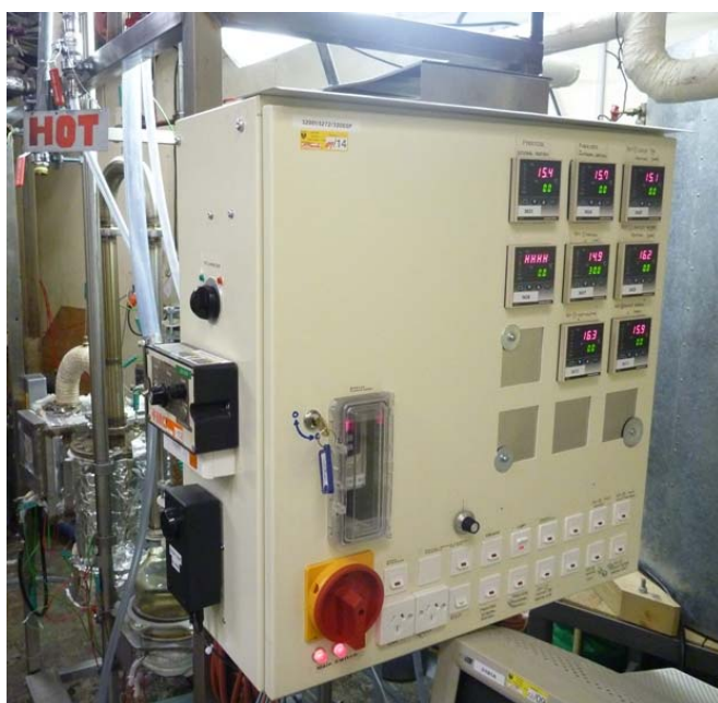
Figure 7-12 Control panel of the apparatus
