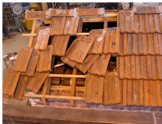
Figure 9: Scattering and falling of unsecured tiles (tied up tiles did not slide)
