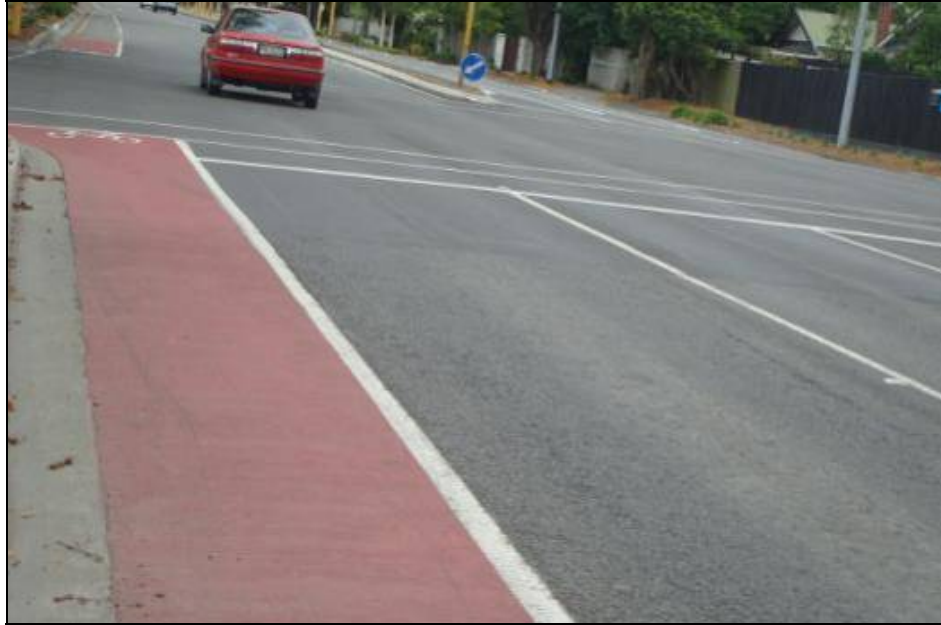
FIGURE 1 Typical Advanced Stop Line (ASL) in Christchurch, NZ
