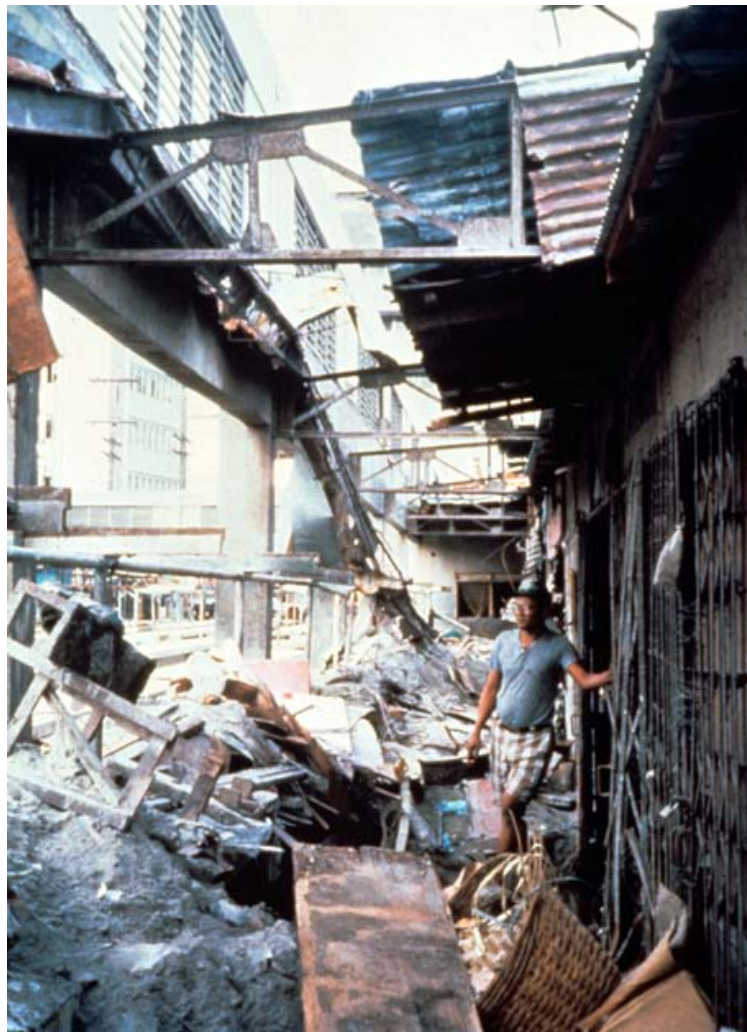
Figure 10 – Rain-saturated ash from the 1991 eruption of Mt Pinatubo in the Philippines collapses a roof in a public market (photo: T. J. Casadevall U.S. Geological Survey).
