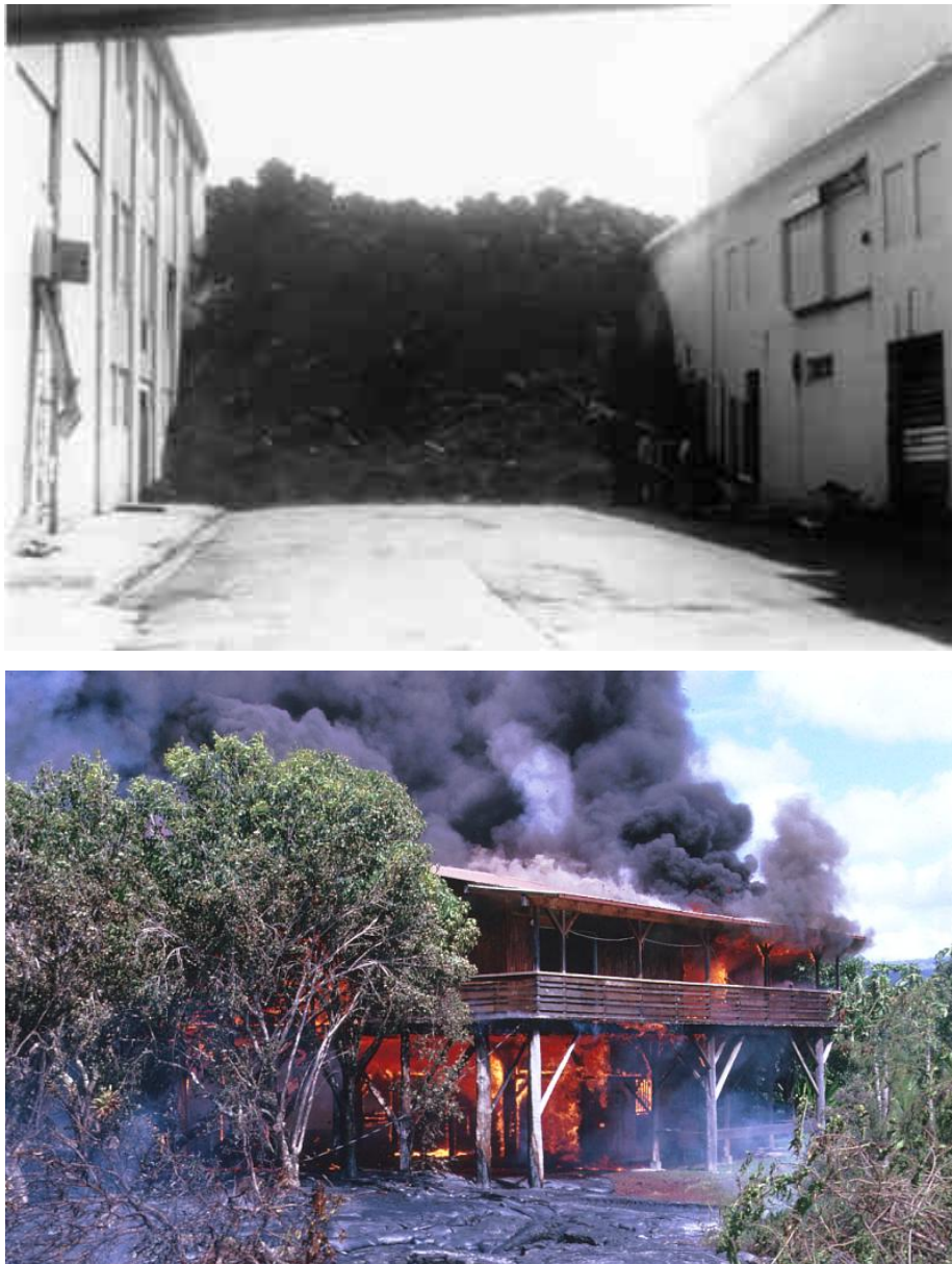
Figure 8 – The masonry buildings of Heimaey (above) withstood the lavas onslaught and were able to be restored to use within a year of the 1973 eruption. Wooden homes in Kalapana, Hawaii were completely incinerated when the thin lava fronts entered their communities, during the extended eruption of Kilauea (photos: HVO 2007).
