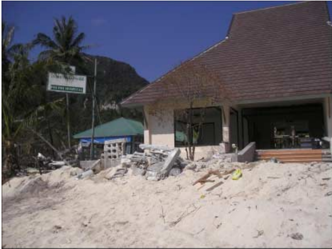
Figure 8. The hospital on Koh Phi Phi was set back from the shore but situated close to sea-level. It was rendered inoperable by the tsunami, highlighting the critical need to locate such facilities outside potential inundation zones (Photo LY).
