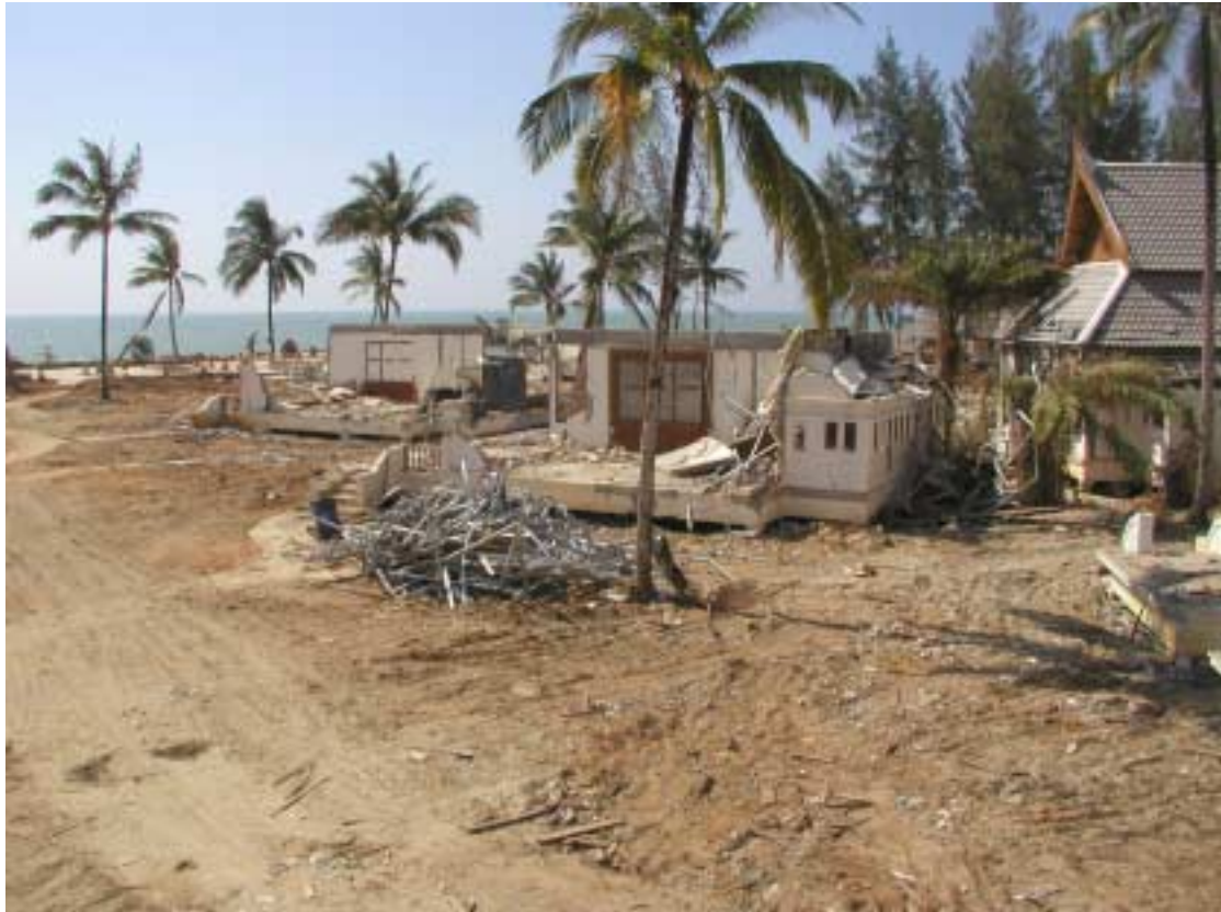
Figure 11. View to seaward at one of the coastal resorts in Khao Lak. Foundations are all that remains of the single-storey buildings closest to the beach. A gradation in the severity of damage owed more to the protection afforded by adjacent structures than to the absolute distance inland (Photo HC).
