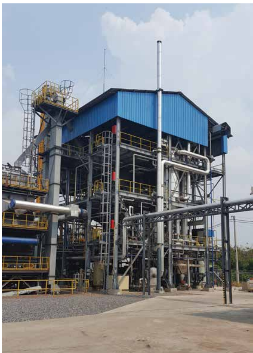
Nongbua dual fluidised bed biomass gasification plant (1 MW electricity, 4 MW biomass input) in Nongbua, Thailand, which uses Güssing Renewable Energy Co. Ltd technology
