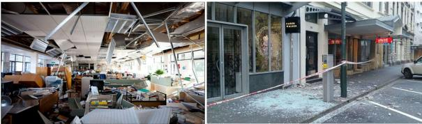
Figure 1: Illustrating damage to non-structural elements observed in the Canterbury earthquakes (left, from Dhakal, 2010) and Kaikoura earthquake (right, from Radio NZ/Susie Ferguson).
