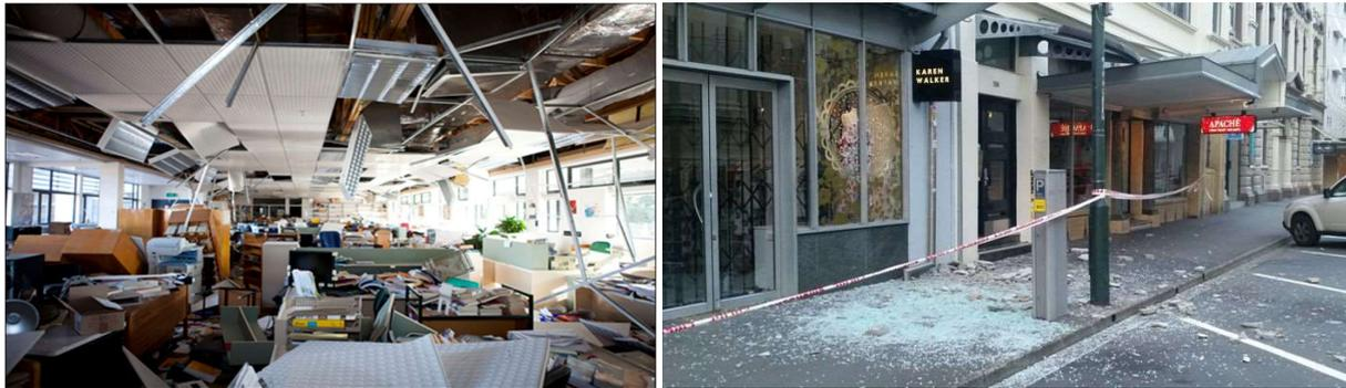
Figure 1: Illustrating damage to non-structural elements observed in the Canterbury earthquakes (left, from Dhokal, 2010) and Kaikoura earthquake (right, from Radio NZ/Susie Ferguson).
