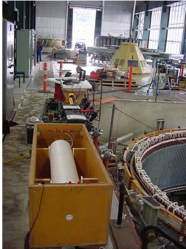
Figure 2 Resonant Inductor in use at Matahina
