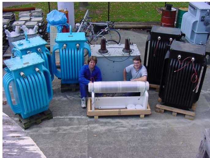
Figure 6 Manapouri Resonant Transformer in front of Equipment Previously used at Tekapo Power Station.
