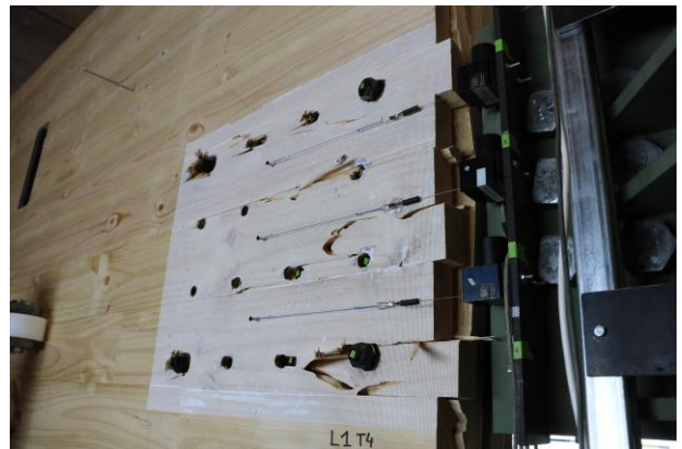
Figure 12: Failure of connection 04
