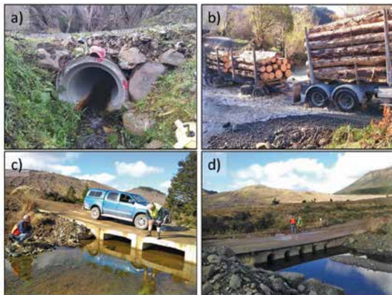
Figure 1: Stream-crossing types included in the field survey of road design, water control and surface cover BMPs: a) single culvert; b) open ford; c) drift deck; d) battery culvert
