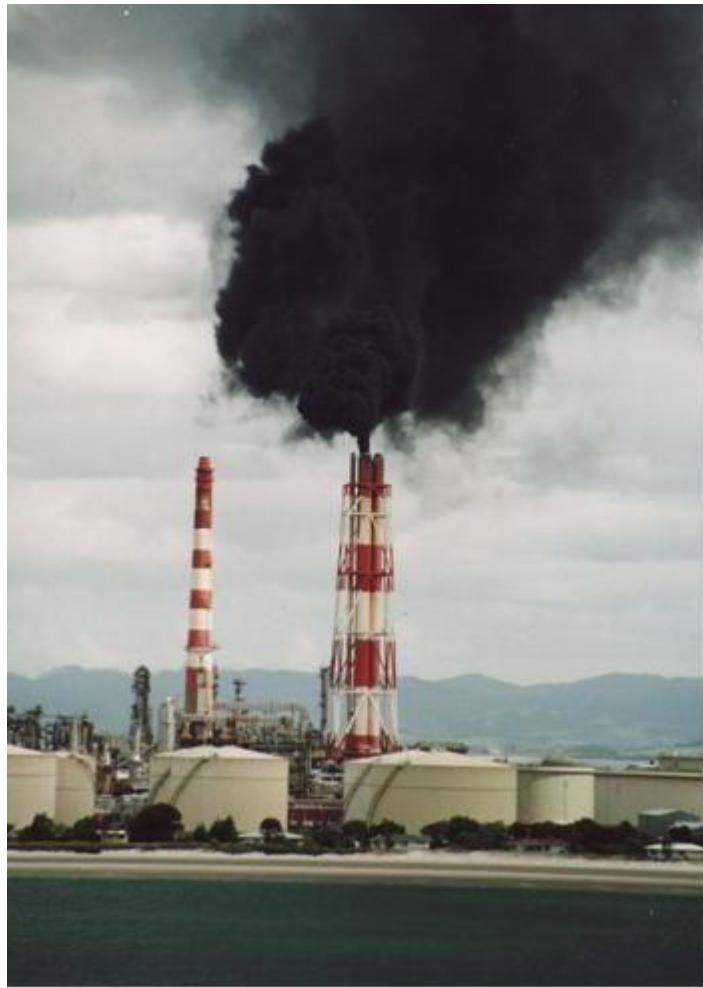
Figure 5.20 ‘Minor process upset’ at the New Zealand Refining Company - 2005 (photograph supplied by Northland Regional Council).
