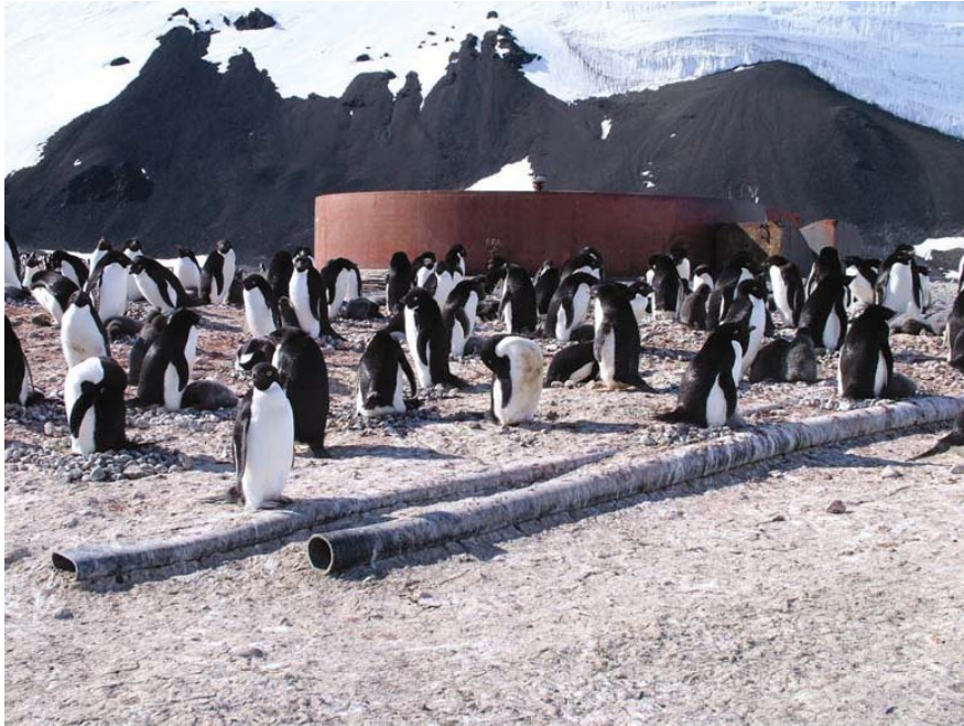
FIGURE 8: PHOTO OF THE BULK (100,000 GALLON) FUEL TANK AT CAPE HALLETT IN 2001. COURTESY OF THE ANTARCTIC TREATY CONSULTATIVE REPORT 2006
