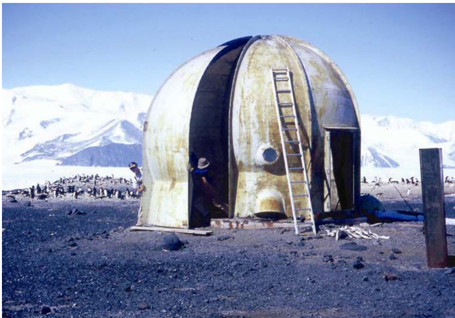
FIGURE 9: THE GEOMAGNETIC DOME BEING DISMANTLED ON SITE AT CAPE HALLETT. COURTESY OF ANTARCTICA NEW ZEALAND
