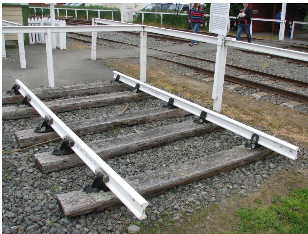
Figure 7. Section of recreated broad gauge track with double head rails at Ferrymead Heritage Park, 24 October 2016. Photograph: A. A. Cross.
