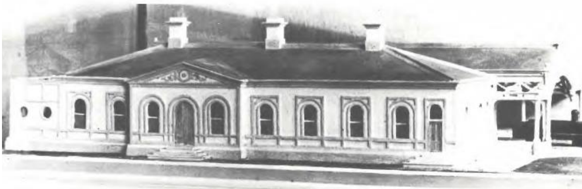
Figure 25. Model of the 1864 Invercargill Station, as built by the Oreti Railway. Model of steam locomotive N o 2 protruding from decorative end of train shed at right. Photograph: Mahoney, p.
