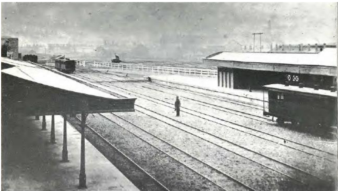
Figure 24. Platforms 1 and 2 at the Christchurch Railway Station, 1878. Additional carriage sidings and passing tracks between platform lines, with at least three 'C'-class six-wheel narrow gauge carriages present. Photograph: Pierre, p. 100.
