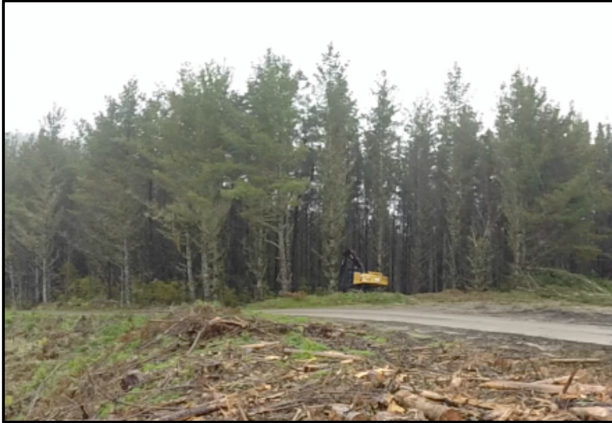
Figure 4: Site 3, the area where all mechanised felling into the stand took place on a slope of 38%.
