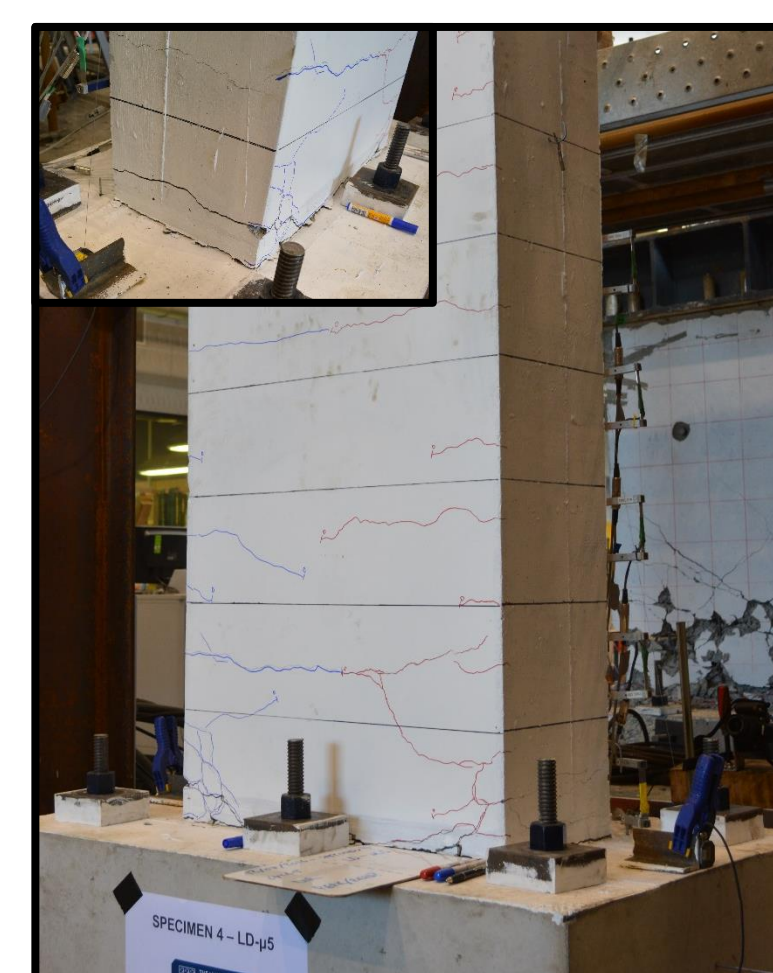
Figure 3: Damage state following dynamic long duration EQ loading to ductility 5, with close up of primary and bond splitting cracks in inset.
