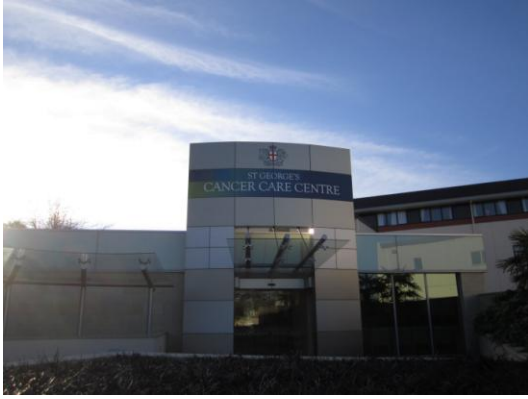
Figure 3.9: St George's Hospital Cancer Care Centre
