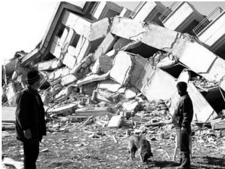
Figure 1.1: Devastating effects of 2002 Afyon Earthquake (M=6.2) on a residential concrete building.
