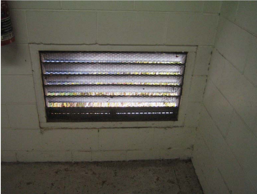
Figure A2.4: Wall opening in a distribution station
