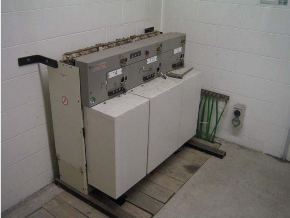
Figure A2.2: Oil insulated high voltage switchgear
