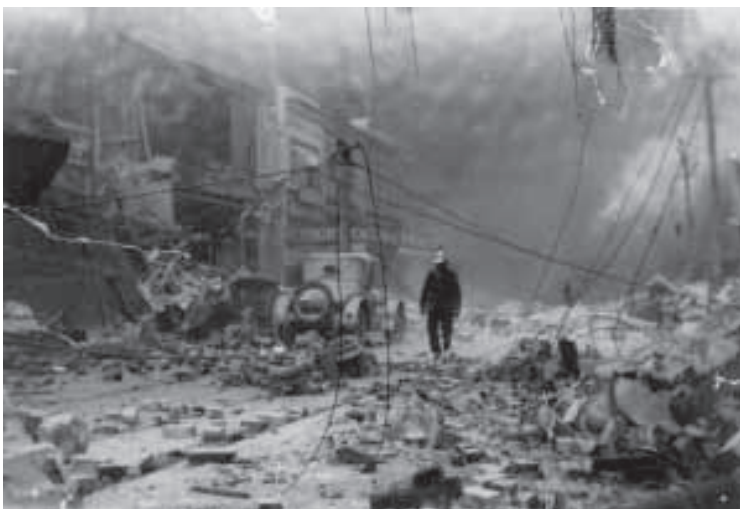
Debris in streets creates difficulty in access for firefighters after the Napier Earthquake, 1931 (photo courtesy of The National Library of New Zealand)
