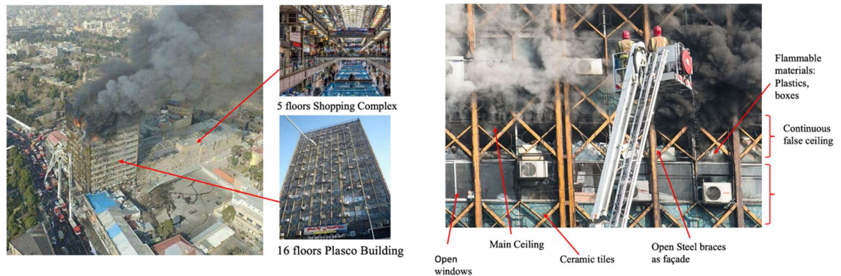
Fig. 2: Detail of the Plasco Building 31,32
