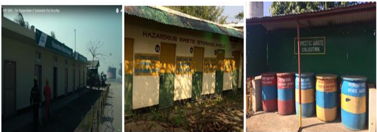
Figure 4.10 Photographic evidence of High, Medium & Low level of Hazardous Waste Storage
