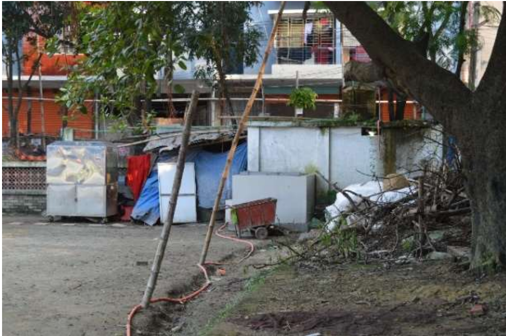
Figure-4.8: Poor condition of toilets and water supply (Ward 33)
