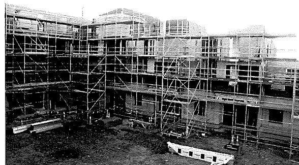
Figure 1: Multi storey rest home in Cross Laminated Timber
