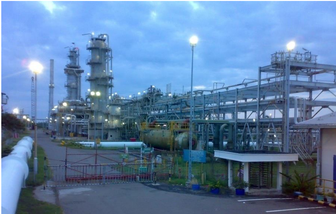
Photo 3-1 Arun ExxonMobil site in Lhoksukon, North Aceh
