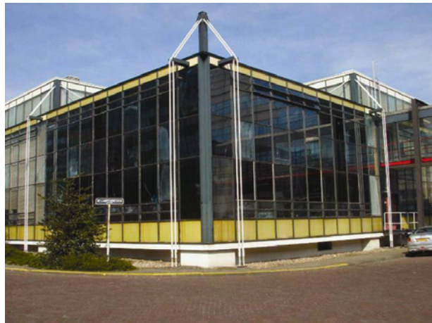
Figure 1 The Alice installation inside the W-hal building (see online version for colours)
