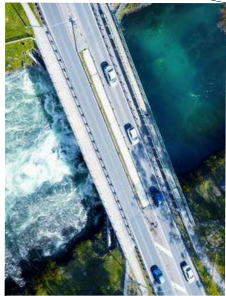
Figure 2.11: Photo of Taupō control gates (Source: Mighty River Power, 2015)
