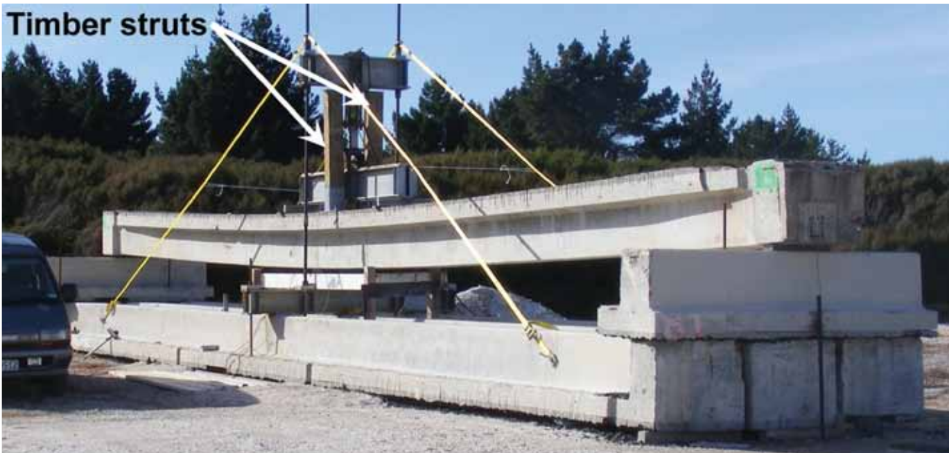
Figure 11. Test rig and deflected good-condition beam.
