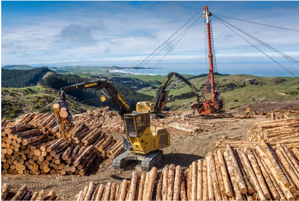
Figure 6.1 Example of a skid operation, where the stems are extracted using the yarder in the background, then cut up into logs and subsequently sorted and stacked for loading out (photo courtesy of Phil Taylor)
