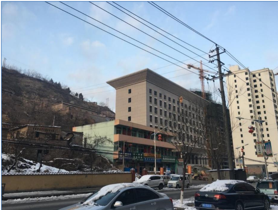
Figure 10 New building replacing yaodong near completion
