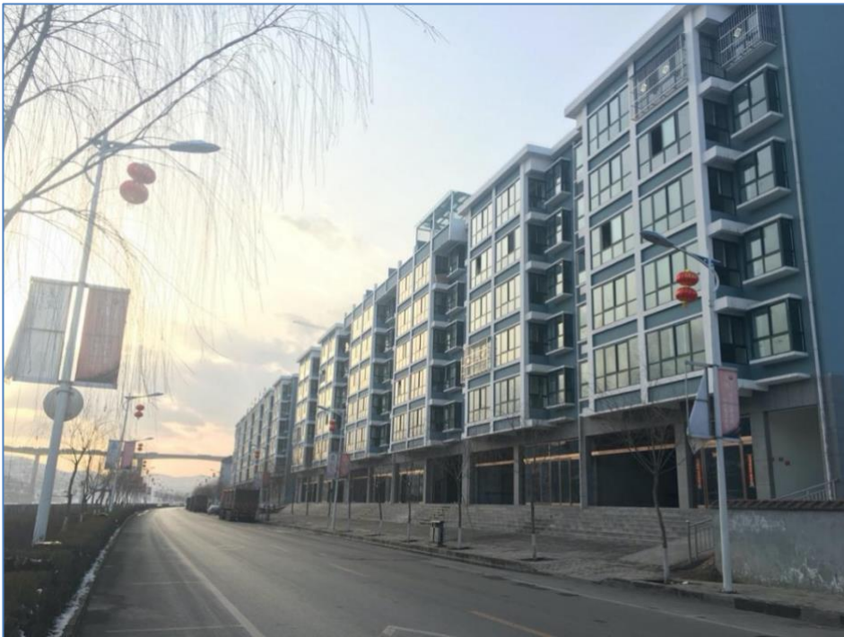
Figure 2 Residential buildings near completion by the Yellow River
