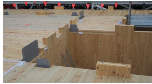
Figure 2: 3-storey CLT structure, Christchurch (c/o EngCo and PTL Structural Consultants)
