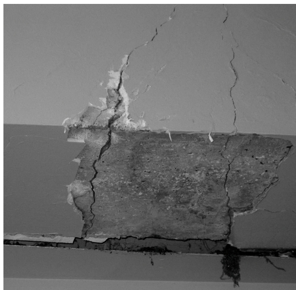
Fig. 5: Cracked beam on Level 8 of the Rutherford Building.
