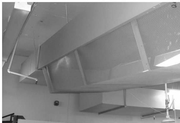
Fig. 4: Ceiling mounted services broke free and finished up resting on sprinkler pipe-work.
