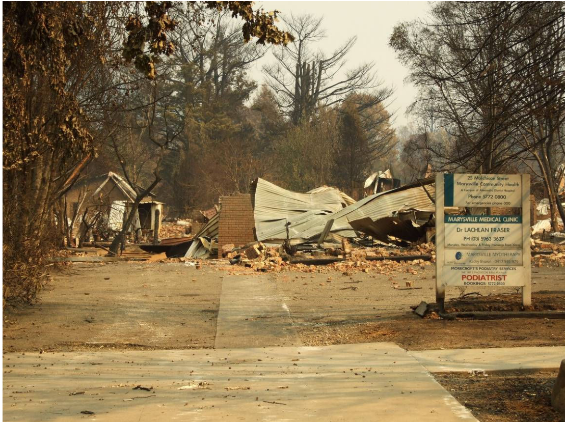
Figure 5.2 The Maysville Medical Clinic before demolition and debris removal (Photo credit: Dr. Lachlan Fraser)
