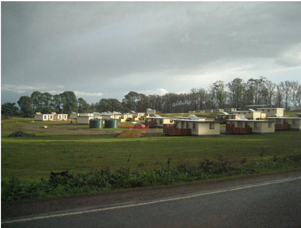
Figure 4.1 Temporary housing complex in Kinglake
