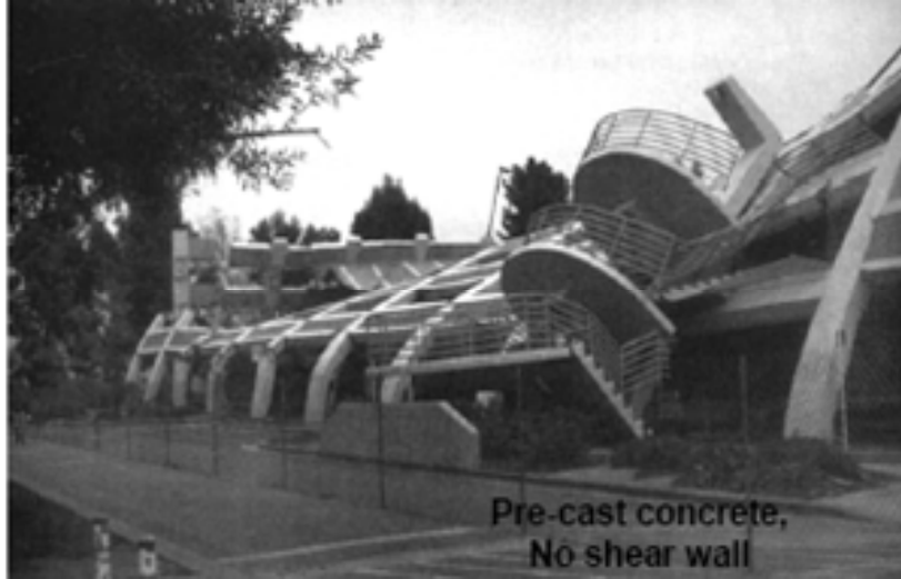
a) Parking Building, California State University, Northridge, 1994
