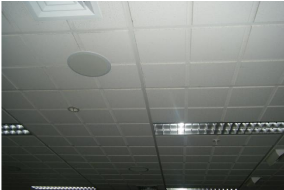
Rare cases of large suspended ceilings with little or no damage (both had light tiles)
