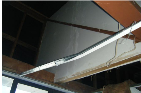
Breaking, buckling and twisting of grid members due to large compression force
