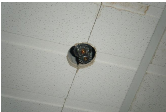
Rigid sprinkler with sufficient gap: no extra damage due to ceiling-sprinkler interaction
