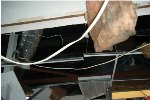
Breaking, buckling and twisting of grid members due to large compression force
