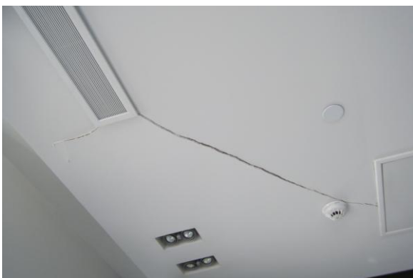
Damage to a plasterboard ceiling in a high rise office building in the city
