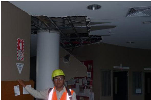
Damage to flush type ceiling in a four story building in Hereford Street
