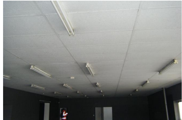
Rare cases of large suspended ceilings with little or no damage (both had light tiles)
