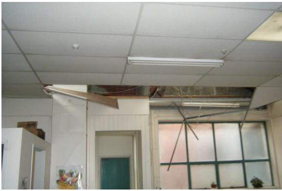
Typical grid failure at the end span near the wall due to accumulated force
