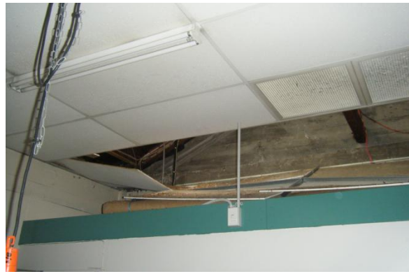
Typical grid failure at the end span near the wall due to accumulated force
