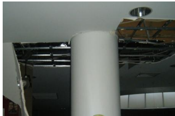
Damage to flush type ceiling in a four story building in Hereford Street
