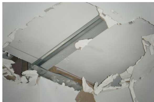
Damage to a plasterboard ceiling in a high rise office building in the city
