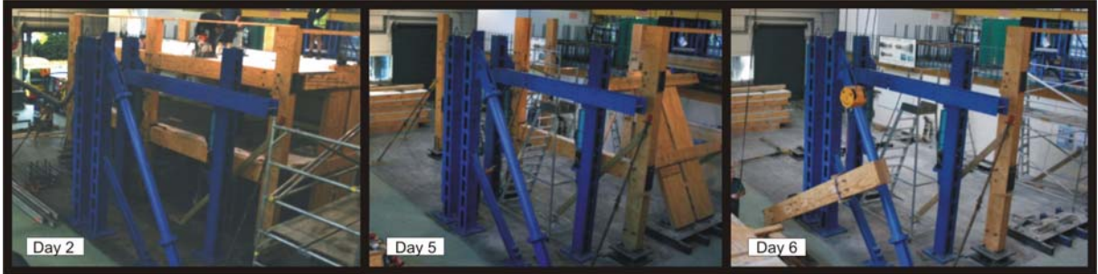
Figure 2. Deconstruction Sequence of Pres-Lam Test Building (Wong 2010)
