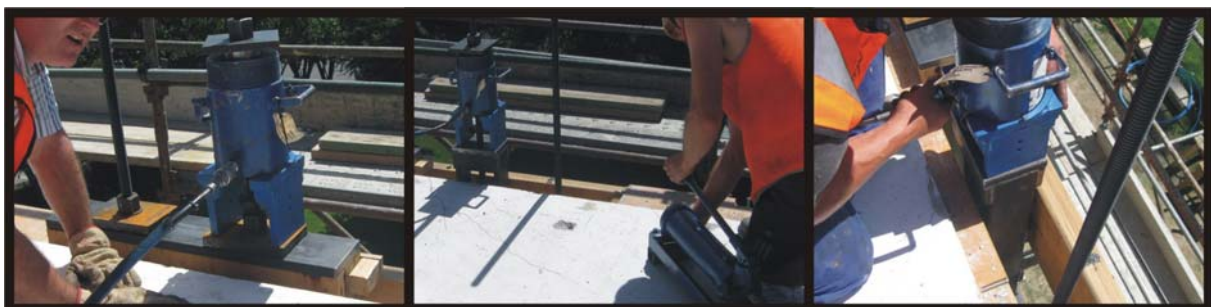
Figure 8 Post Tensioning of the Wall
