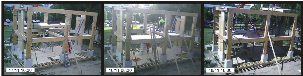
Figure 7. Placement of Floor Units
