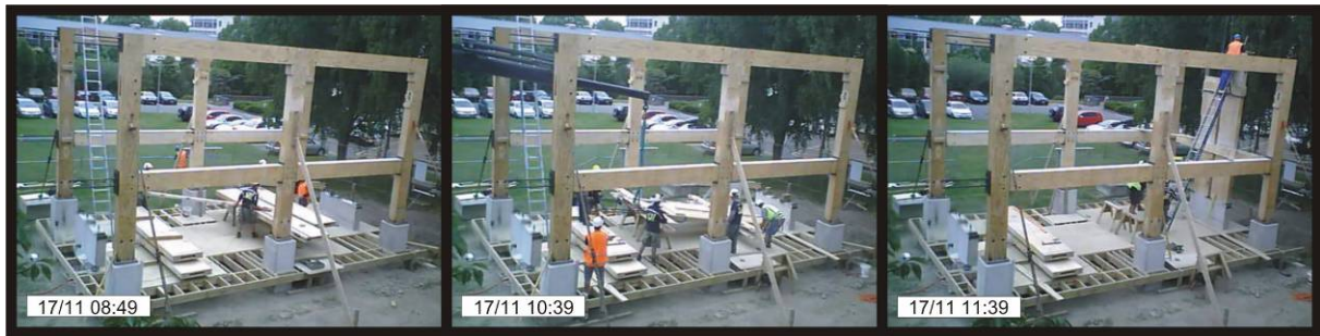
Figure 6. Erection of Post Tensioned Timber Walls
