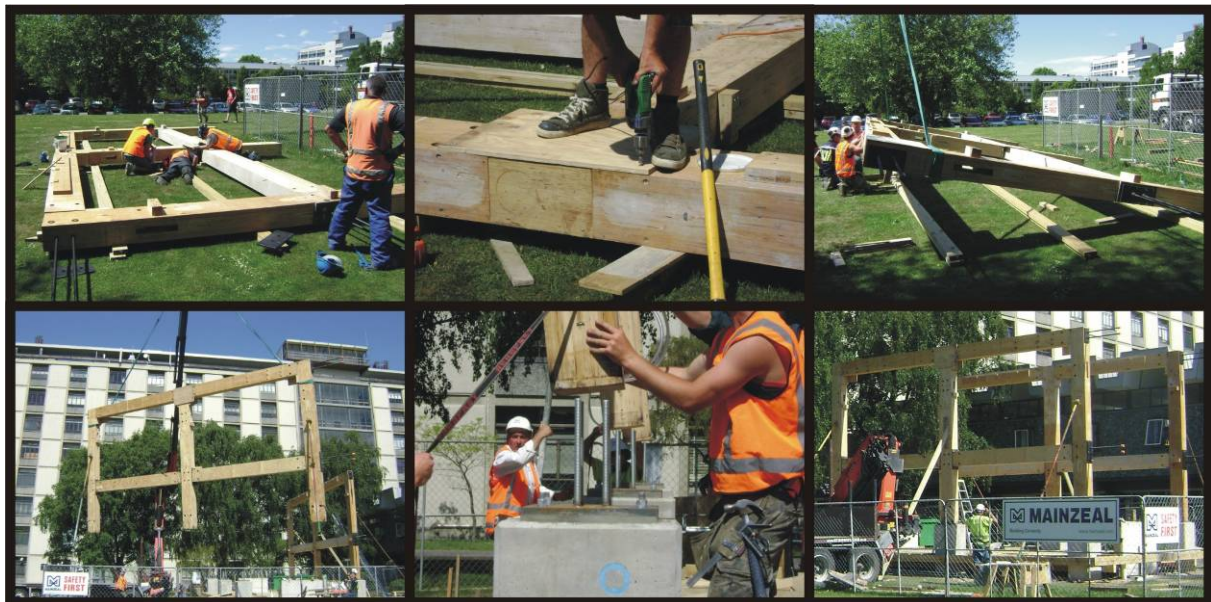
Figure 5. Erection of Second Post Tensioned Timber Frame
